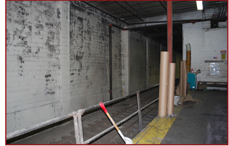
Rail line running through the 1960s warehouse
