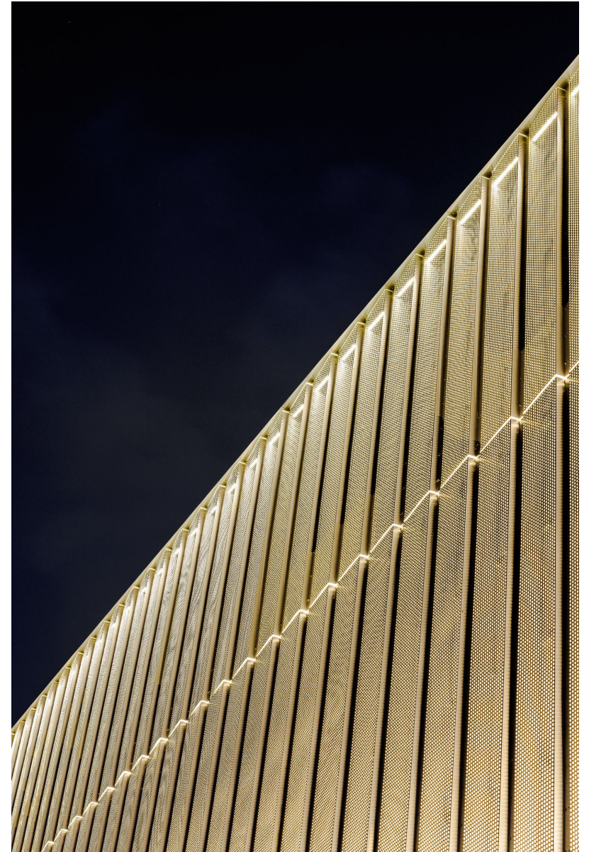
Detail of Wall-wash Light Visible Through Metal Panel Perforations
