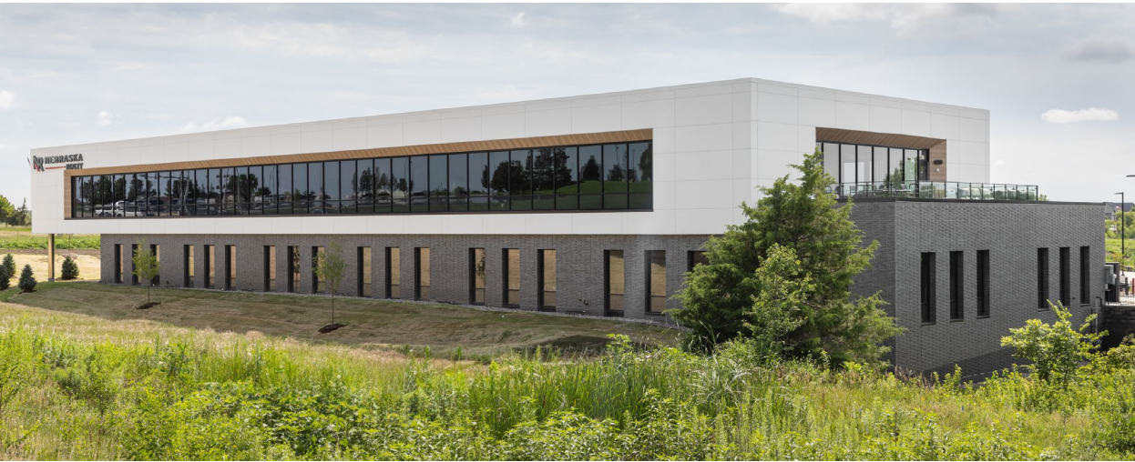
Southwest View from 84 th Street – Formal Shift Creates Roof Terrace
