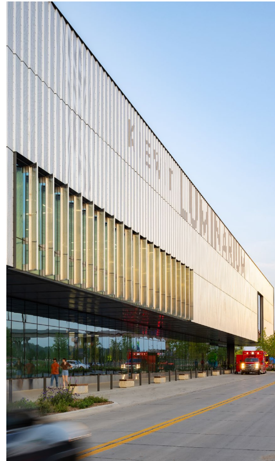
Vertical Sunshades at Second Level Office Suite
