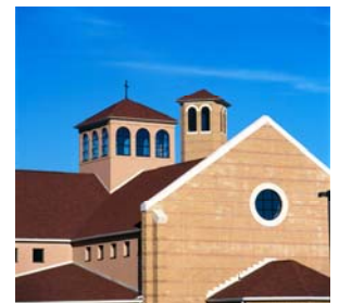
ST. FRANCIS OF ASSISI CHURCH WEST DES MOINES, IA
