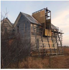
[a] FACT working on Victoria House at Art Farm, Nebraska
