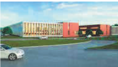
MCC Technology Center
